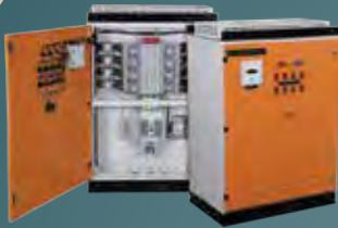
Contactor / Thyristor Switching APFC Panel
