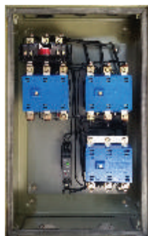
Interior View of ML FASD
