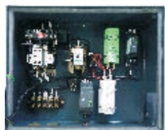
Interior View of MR-G2W
