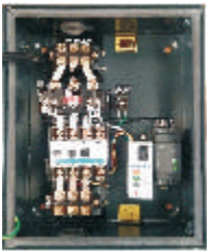
Interior View of MU-G10W DOL
