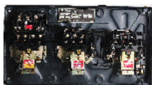
Interior View of MK1 FASD
